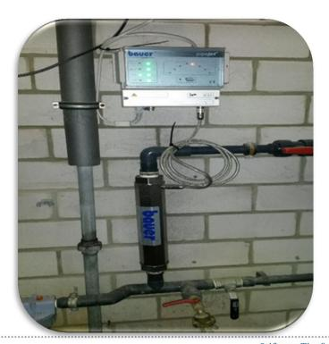
Drinking water is treated by an varied-frequency magnetic field. This field changes crystalline structures (e.g. calcite to aragonite) and should reduce deposits in pipes.
