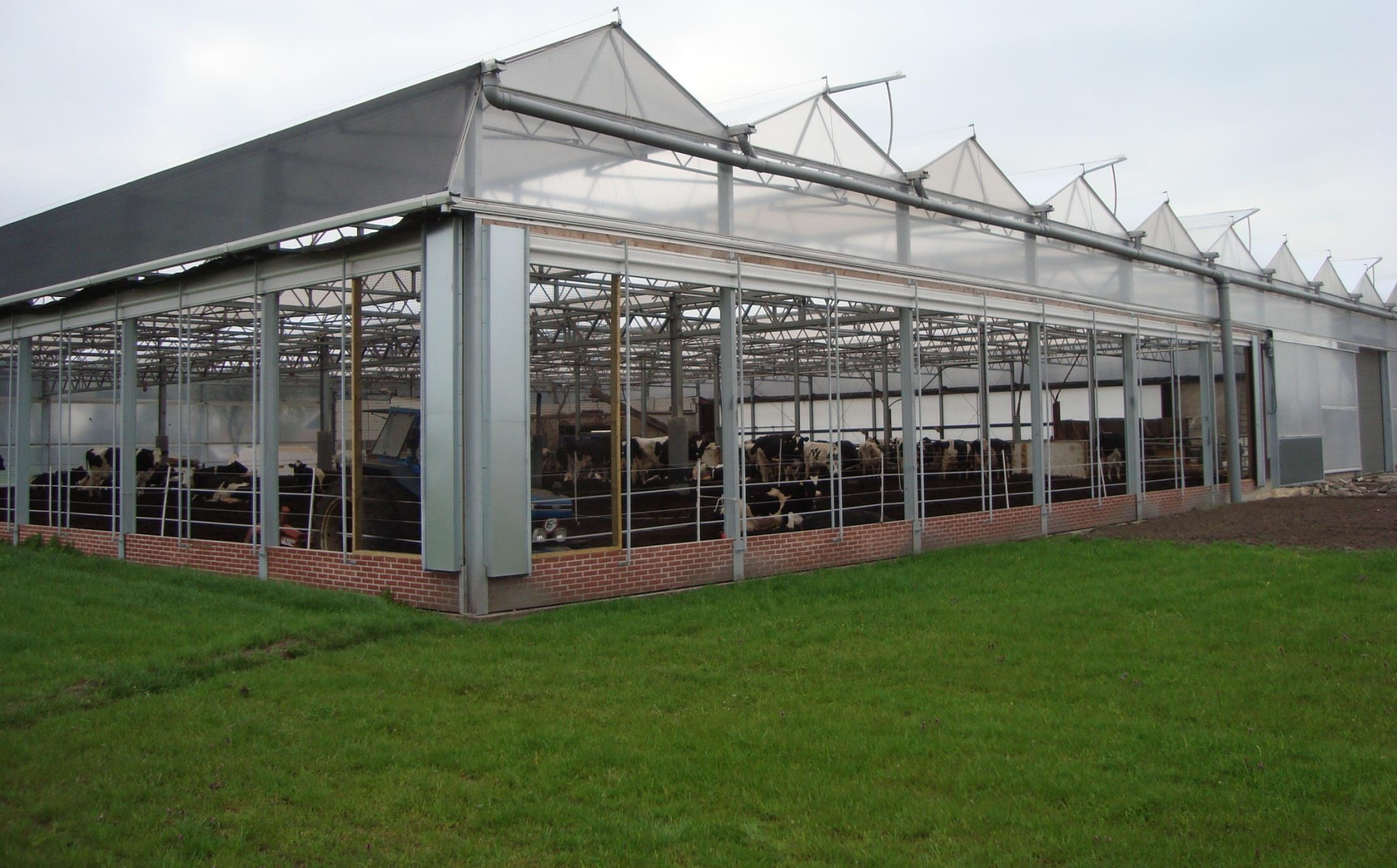
Roof from horticulture
