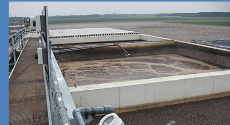
Spreading and treatment
