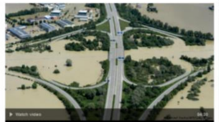
After the flood: A German town in recovery
