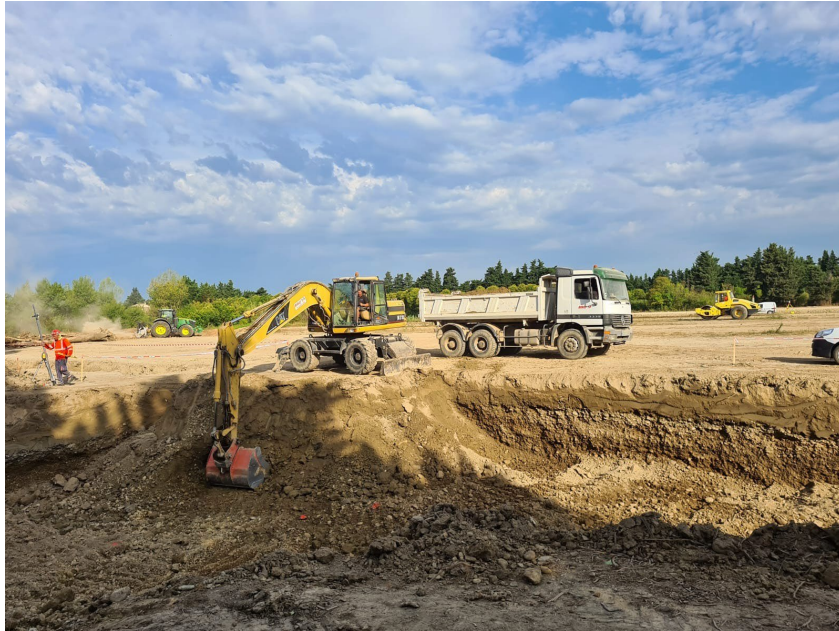
Construction of DEMOTEC, industrial demonstration farm
